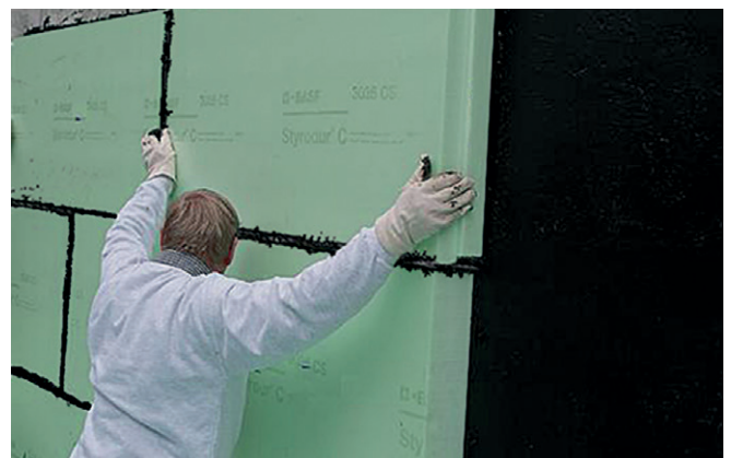
Fig. 17: Setting the Styrodur boards and sealing the joints against pressing water.
