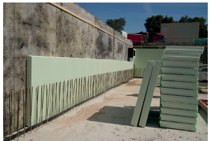
Fig. 30: Installation of Styrodur Hybrid on the inside of the formwork
