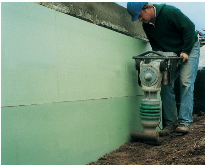
Fig. 29: Mechanical compacting
