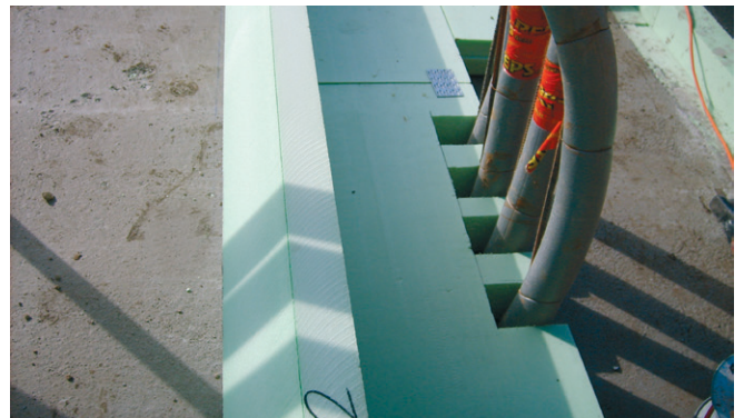
Fig. 42: Cut-outs or penetrations are dimensioned according to structural requirements and local conditions. Any remaining cavities are sealed with special PU foam.
