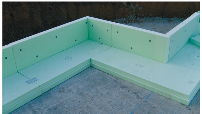
Fig. 36: The custom-fit pre-made and numbered corner elements kit ensures that the edge elements are laid with millimetre accuracy even with structured building footprints. This eliminates the time-consuming measuring and setting of the floor slab.
