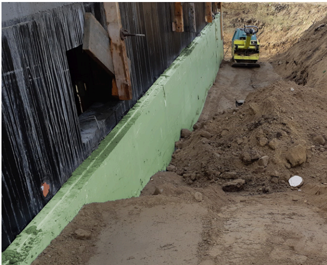
Fig. 28: Layered backfilling
