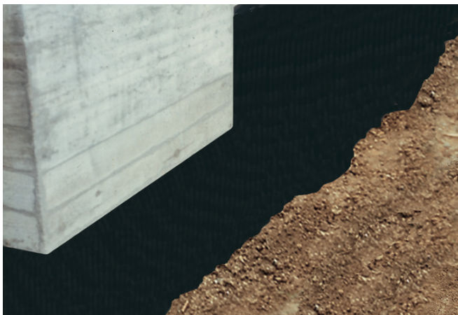
Fig. 15: Waterproofing the basement walls against pressing water.
