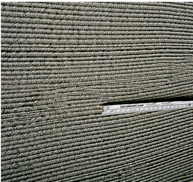
Fig. 24: Horizontally combed bonding bridge on Styrodur insulation.
