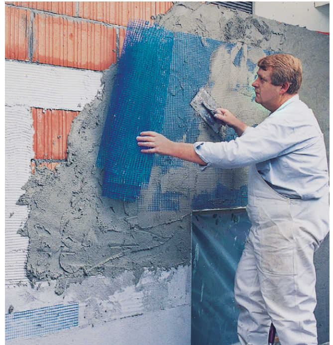
Fig. 22: Application of floating and glass fibre reinforcement mesh on top of insulated concrete elements.
