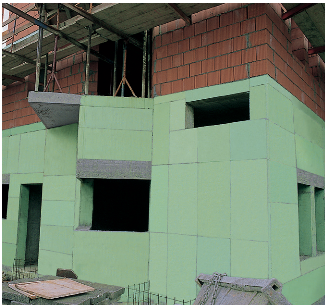
Fig. 25: Large-size ground floor insulation with Styrodur boards.
