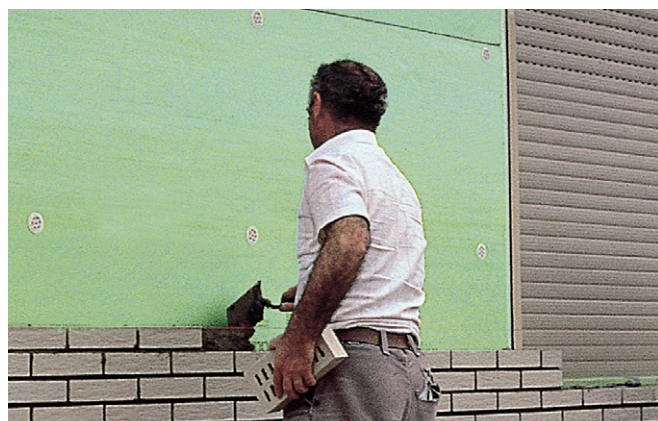
Fig. 33: Cavity insulation with face masonry bricks that are 9 cm wide.
