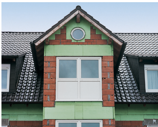
Fig. 1: Thermal bridge insulation of concrete building elements: – Verge – Roof ridge – Ring beam – Window lintel – Ceiling edge
