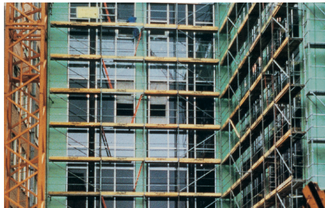
Fig. 7: Thermal bridge insulation with Styrodur 2800 C/Q.
