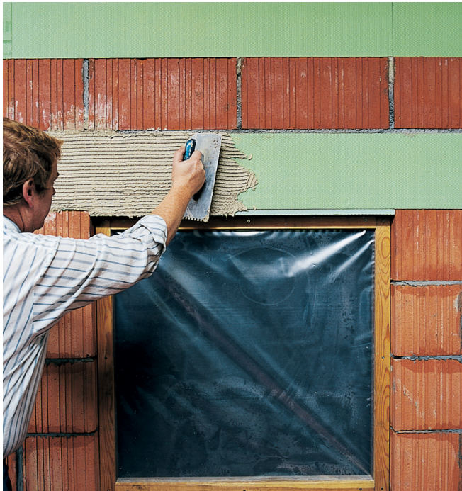
Fig. 20: Window lintel in thermally insulating brickwork; horizontal combing of the plaster bonding bridge.
