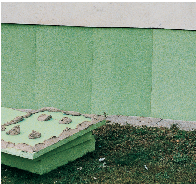
Fig. 31: Renovation of old building: installation of Styrodur 2800 C/Q boards using a dot-bead method.
