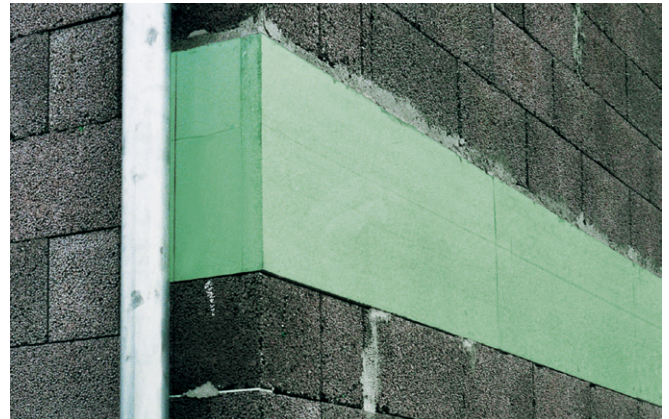
Fig. 2: Thermal insulation with Styrodur 2800 C/Q on the ceiling edge.
