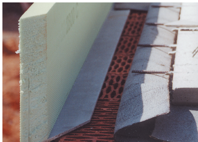
Fig. 8: Ceiling edge formwork with Styrodur 2800 C/Q.
