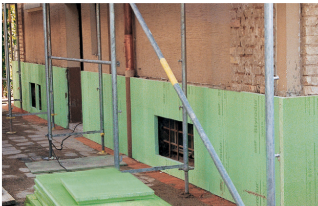
Fig. 17: Subsequent base insulation with Styrodur 2800 C/Q.
