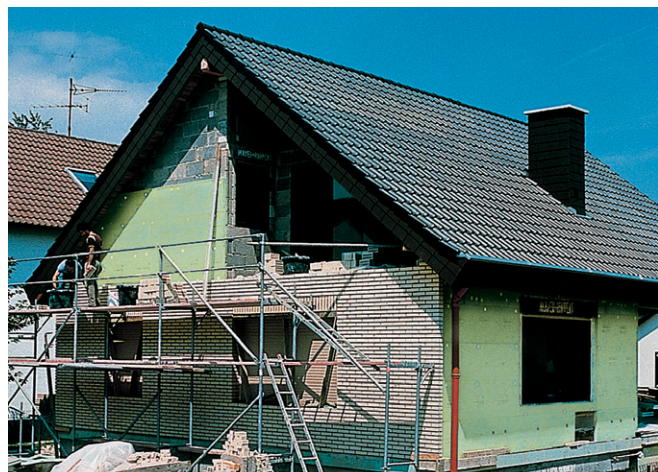
Fig. 34: Cavity insulation with Styrodur.
